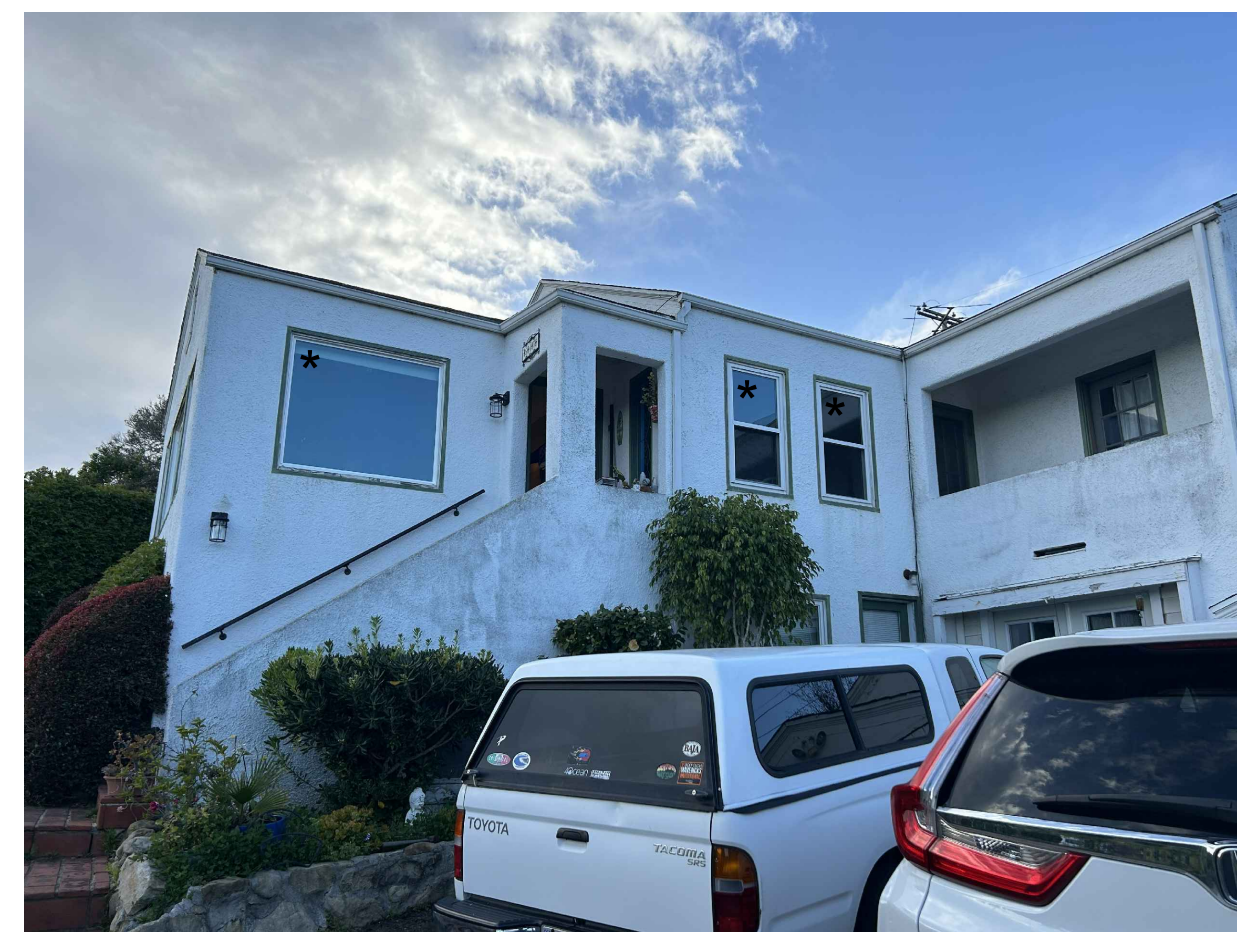
STREET VIEW - LOCATION OF VIYNL WINDOWS
